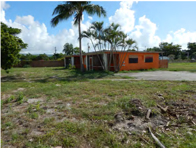
8PB17123_c Facing Northeast
