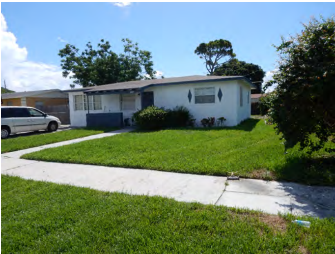
8PB17130_c Facing Northeast
