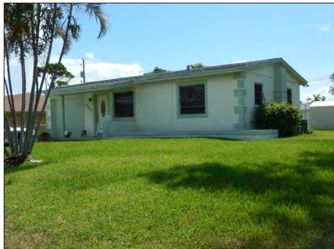
Figure 9. Resource 8PB17131 is an example of a Ranch style building within the project APE. Photograph facing northeast.
