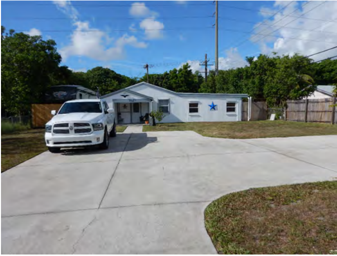
8PB17122_a Facing South
