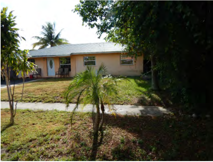
8PB17119_a Facing Northeast
