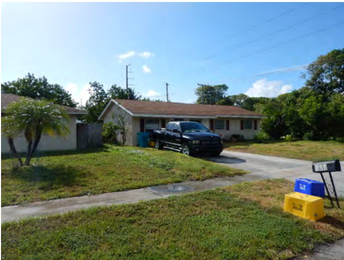
8PB17121_c Facing Southeast
