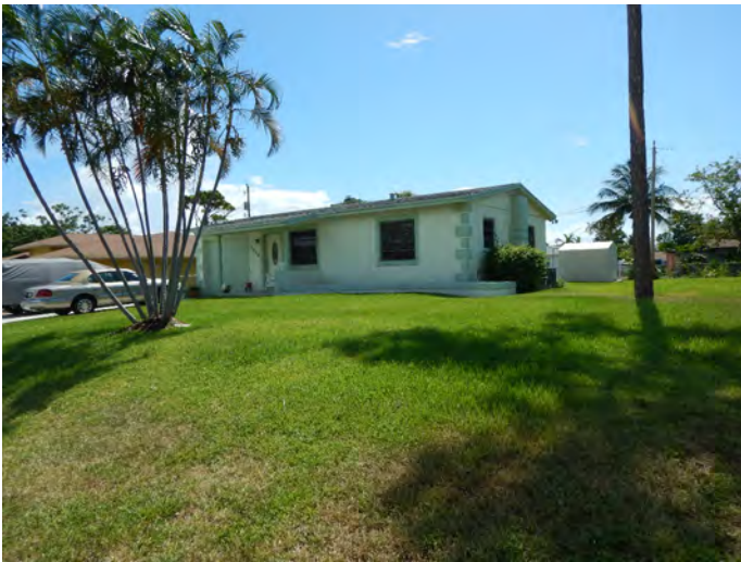
8PB17131_c Facing Northeast
