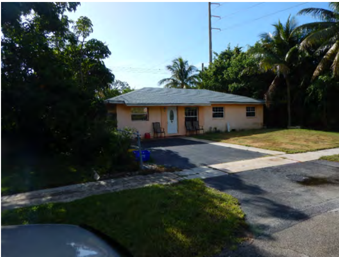
8PB17119_c Facing Southeast
