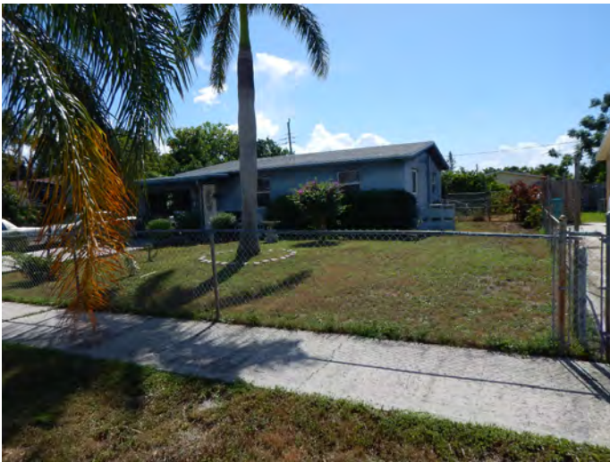
8PB17128_c Facing Northeast
