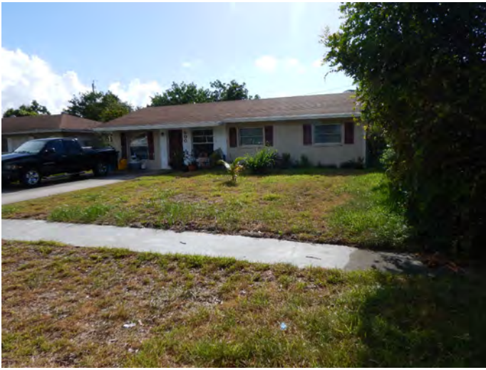
8PB17121_a Facing Northeast
