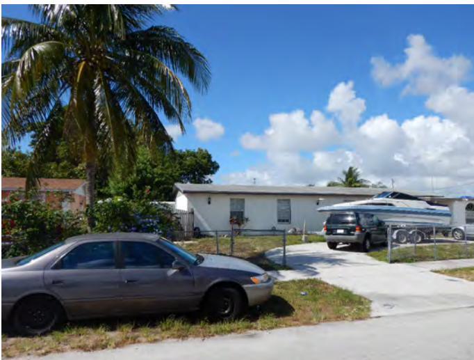
8PB17125_e Facing South
