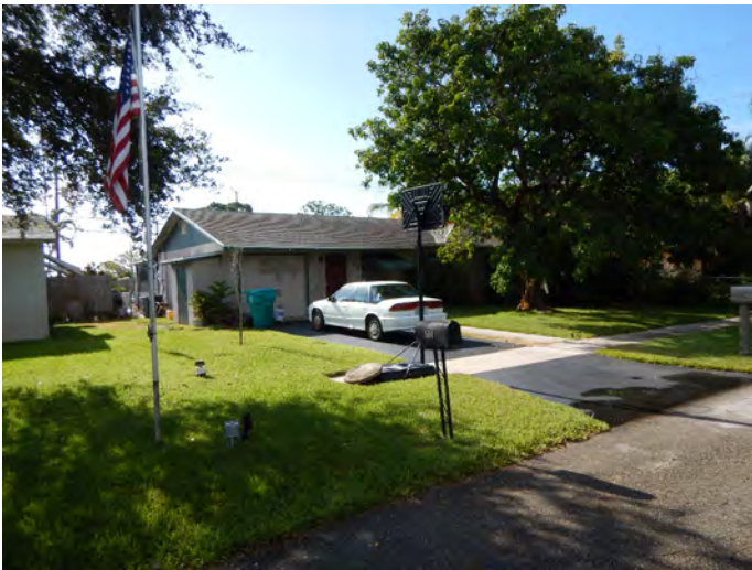
8PB17120_c Facing Southeast
