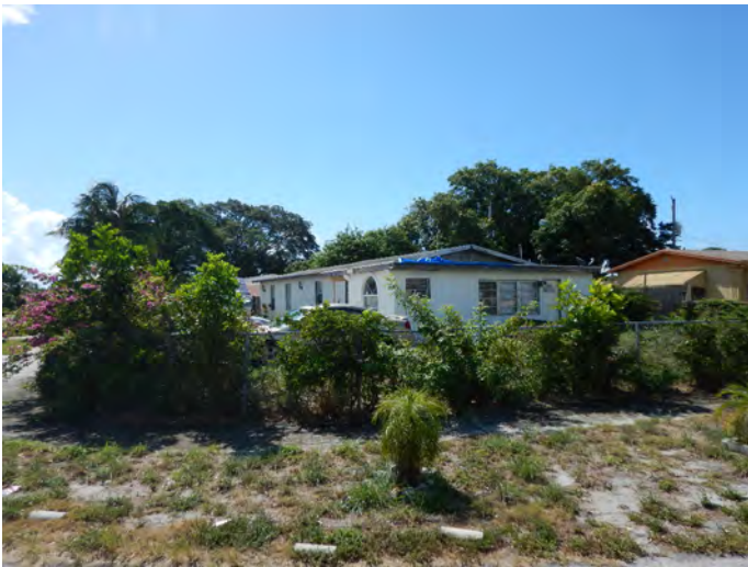
8PB17125_c Facing Southeast
