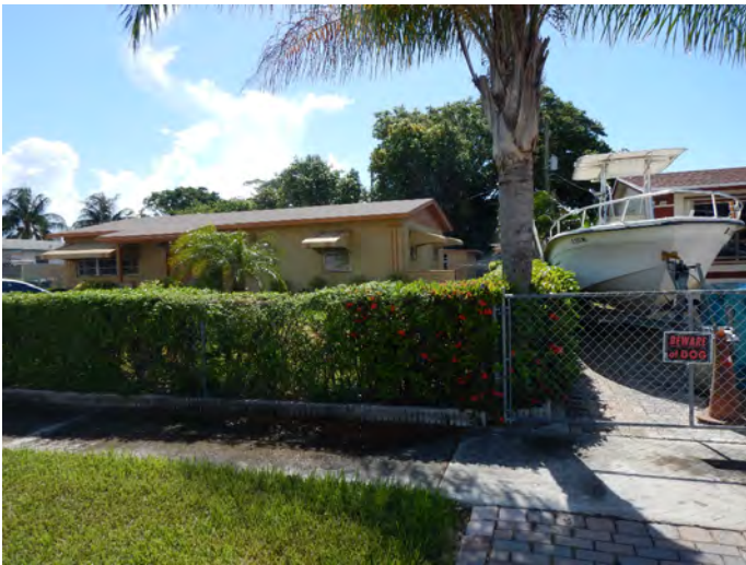
8PB17126_c Facing Northeast
